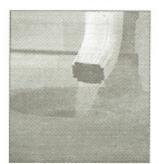
. If you live in regions with heavy rainfall patterns, or have a large area of roof feeding one downsport an additional 45" is recommended to create a "sweep" going directly into the opening.
